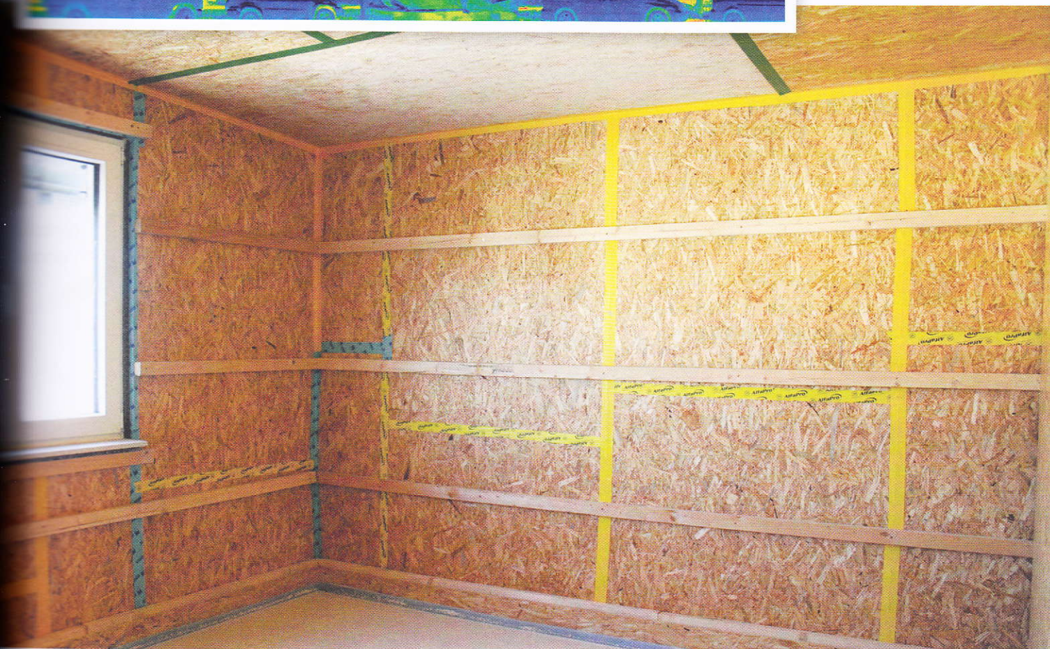
Airtight connectors between wood components in a Passive House under construction. Passive House Institute, Darmstadt, Germany.
